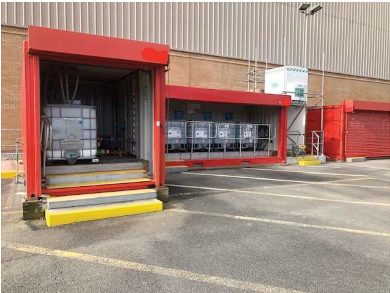
Figure 5: Phase 1 of the Caustic dosing rig with an initial design life initially 10 yrs. Phase 2 will be designed for the life of the facility, is presently in study.
