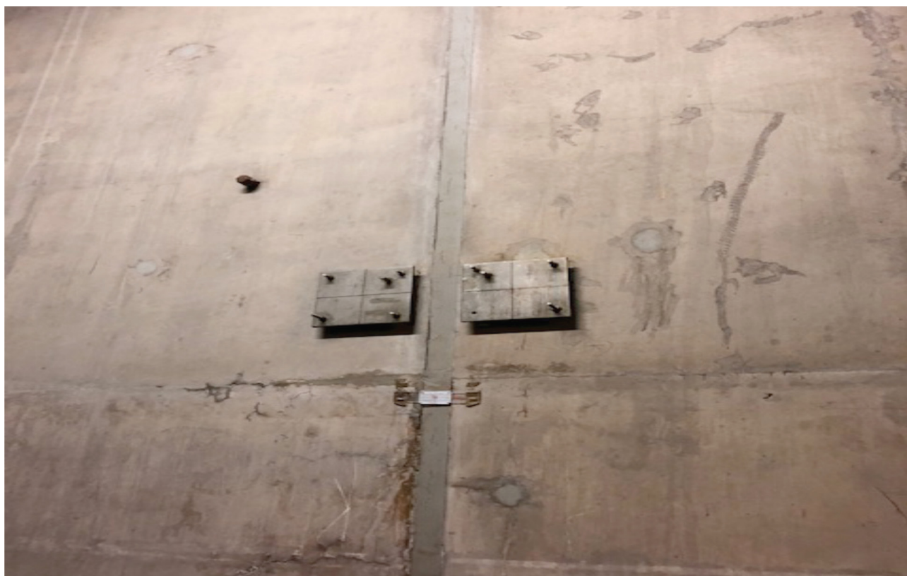
Figure 2: This shows one of the TR&S pond expansion joints with stress and measurement gauges used during an annual engineering system health review. The stub to the left-hand side is a leak detection route that can also be used as part of the repair methodology.
